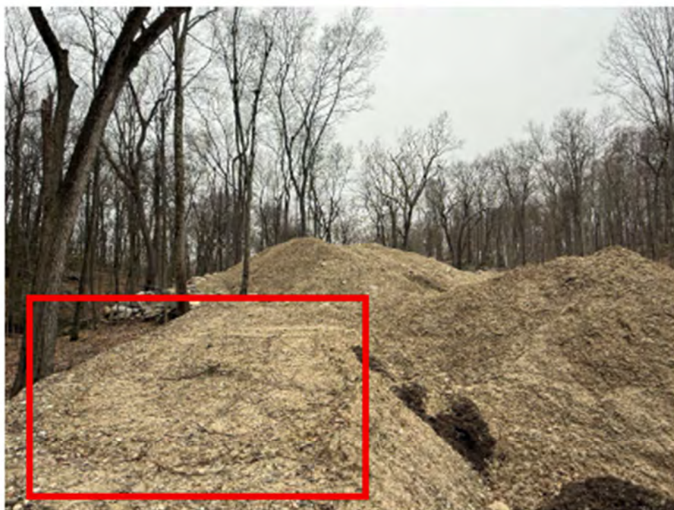
Photo 8: View of the berm area (boxed in red) shown underneath the soil stockpile.
