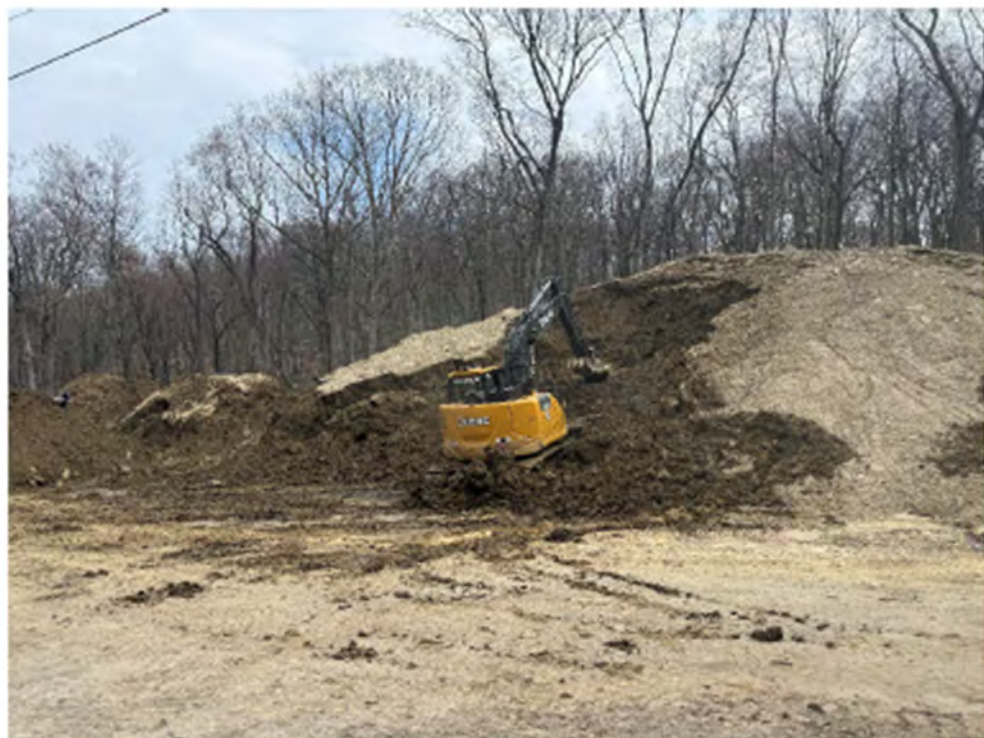
Photo 3: View of excavator working to separate the soil stockpile.
