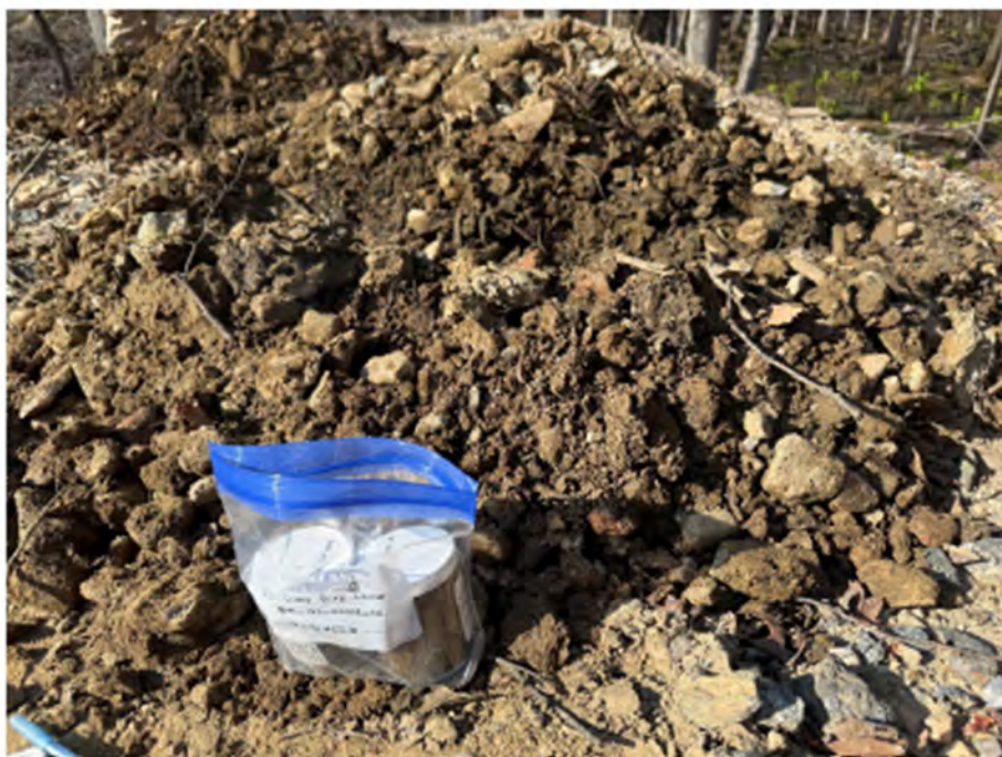
Photo 11: Additional view of berm material with fines, bricks, and concrete.
