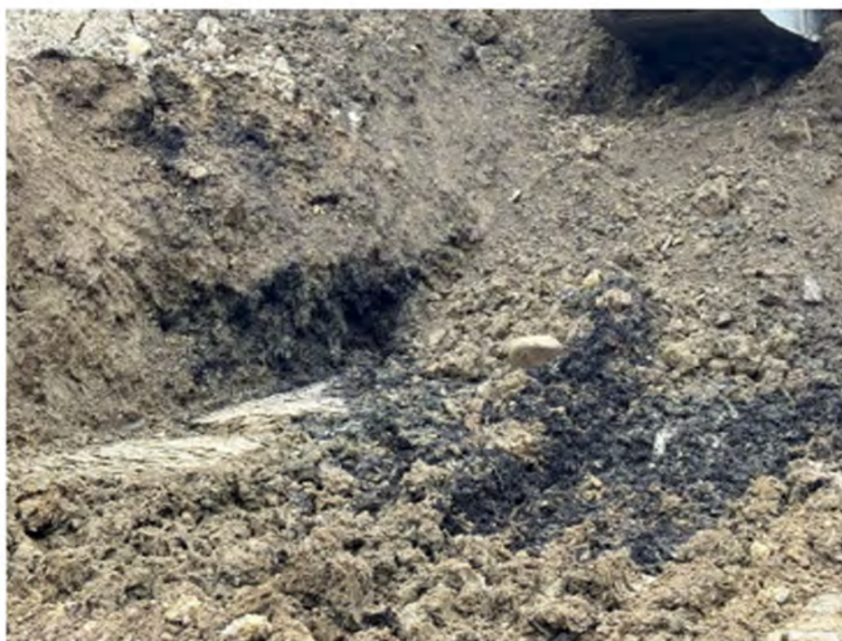
Photo 6: View of suspected mulch encountered while segregating the soil into stockpiles.
